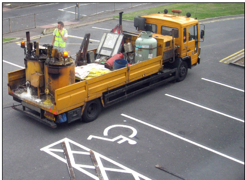
Re-lining front car park – a routine maintenance task for commercial premises – helps to provide hassle-free shopping for visitors to the SRRP site.
