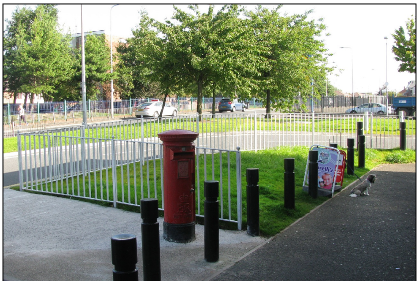
New fencing and landscaping – enhances pedestrian safety, minimises slip hazards, and prevents traffic congestion at the entrance to the SRRP site.
