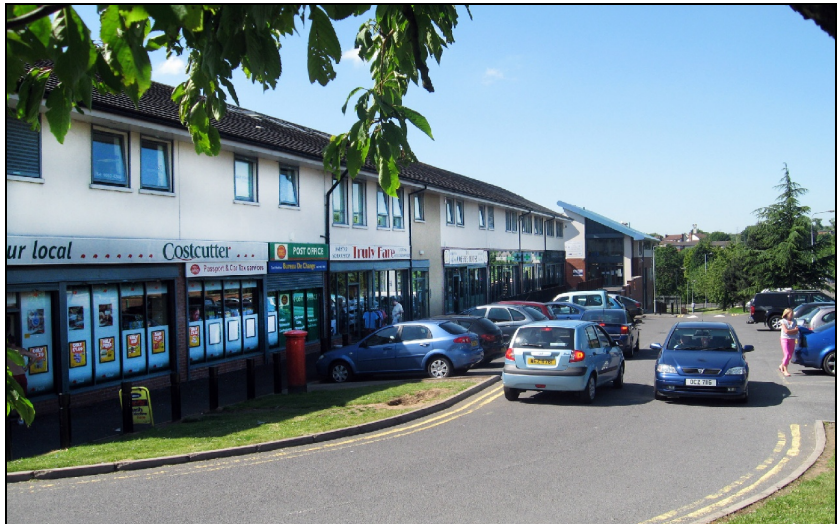
Shops, offices, and children's daycare nursery – a busy hub of activity at the once violent West Belfast, Suffolk / Lenadoon interface.
